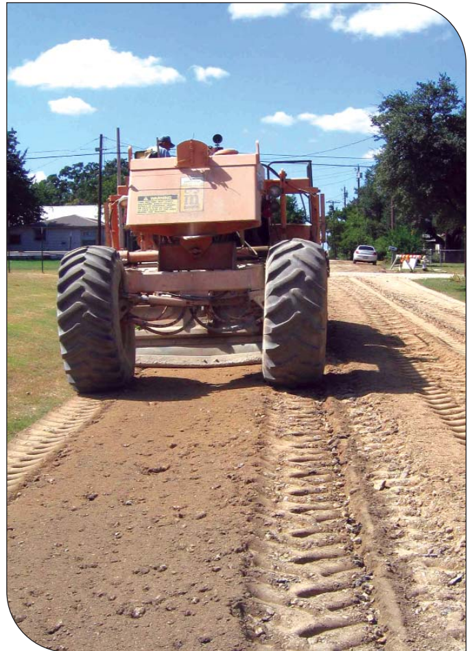
Reclaimer pulverizes the existing street. One or two passes usually achieves gradation requirements.
