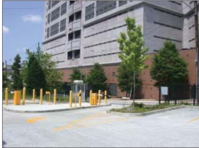
This parking lot built for employees at the Atlanta Bureau of Corrections is constructed with pervious concrete pavement. During most rainfall events, this 55-car parking lot produces no stormwater runoff because rainfall percolates through the pavement and into the soils.
