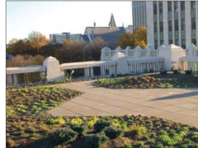
This green roof constructed with donated materials covers part of the fifth floor at Atlanta City Hall. The roof serves as a demonstration of good environmental practice to reduce heat and stormwater runoff and a pleasant spot adjacent to the snack bar for municipal employees to break for lunch.
